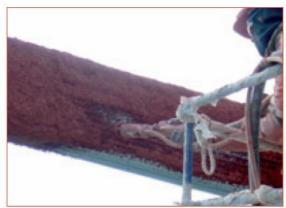
Composed of expanded lightweight aggregate, perlite and vermiculite, hydraulic binders, setting retarders and additives to improve spraying.
